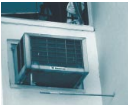
If the aircon projects from the building, it probably needs the stainless steel supports.
